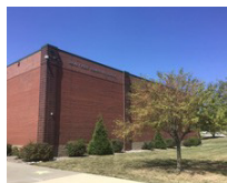
Shoal Creek Elementary
