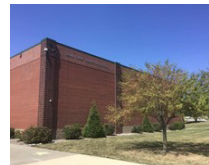
Shoal Creek Elementary
